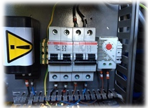
Figure 10 – Isolation MCB's
