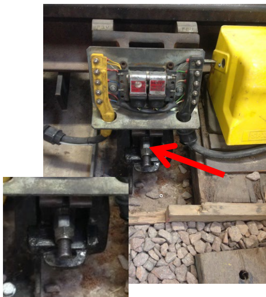
Figure 1 - RCPL and IBCL (with Mk 2 clamp lock) Adjusting Screw field side
