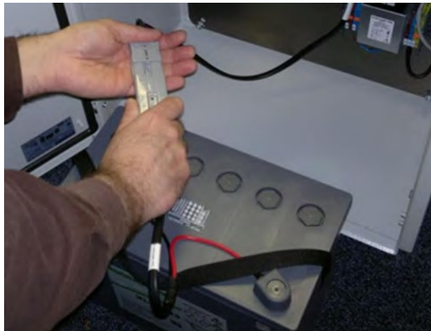
Figure 4 – Battery Disconnection
