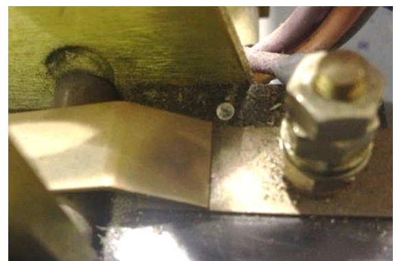
Figure 18 – Cut-out Contact
