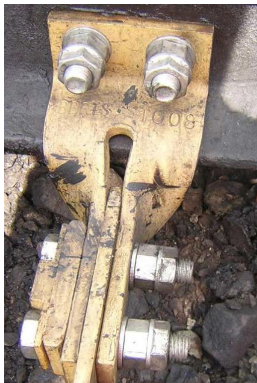
Figure 7 – Yellow stretcher bar bracket with hardlock fastenings
