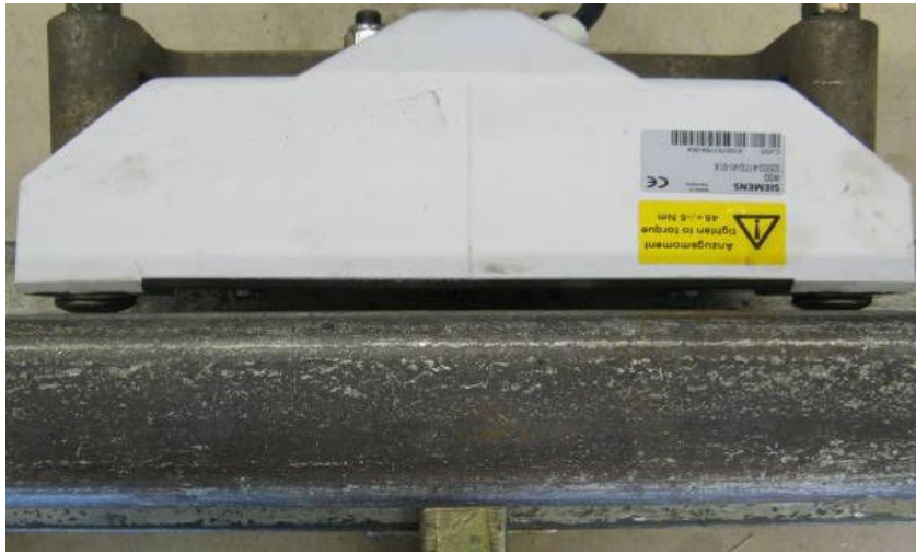
Figure 3 – Too far away from the rail
