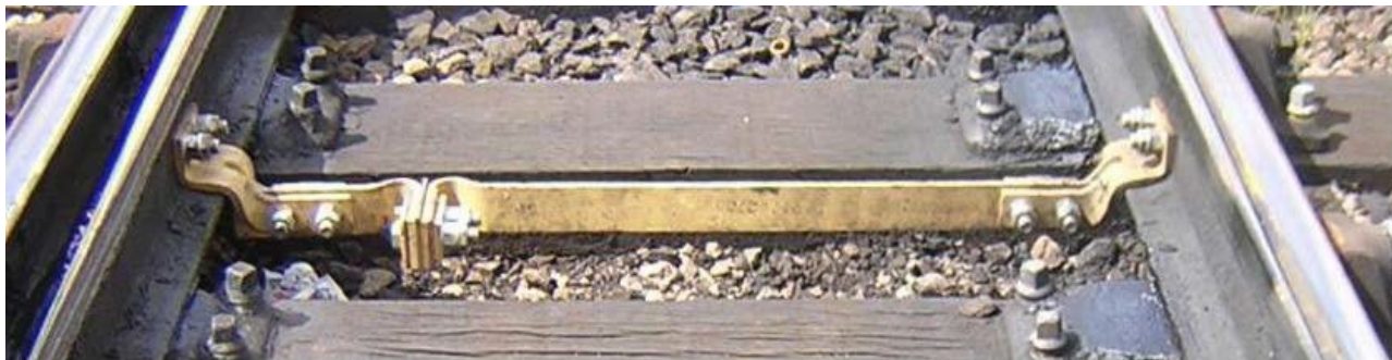
Figure 6 – Yellow fixed stretcher bar with hardlock fastenings
