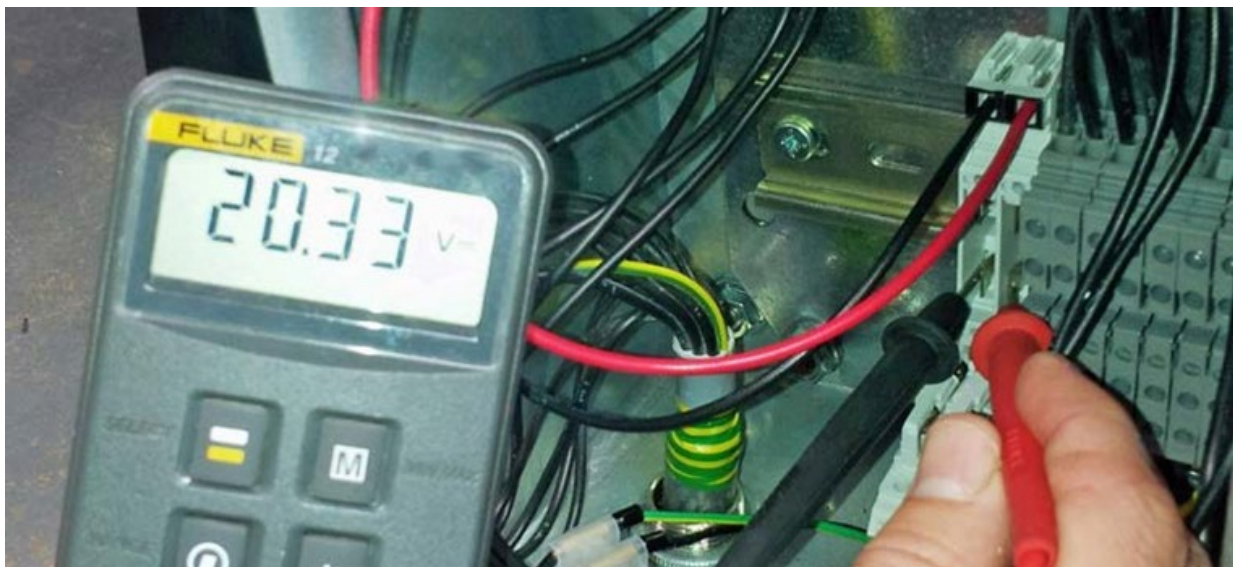
Figure 8 - Solar Panel incoming terminations
