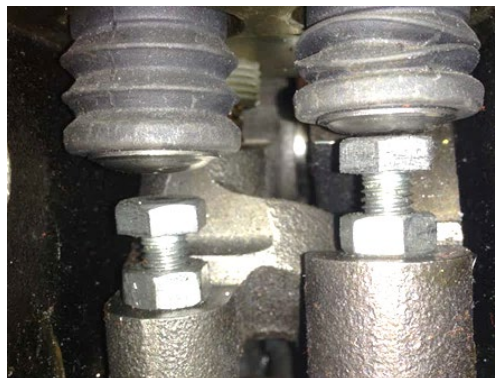
Figure 18 – Micro-switch bellows damage
