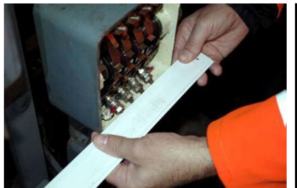
Figure 1 – Stud length check
