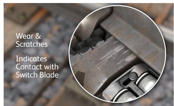
Figure 2 – Check for wear
