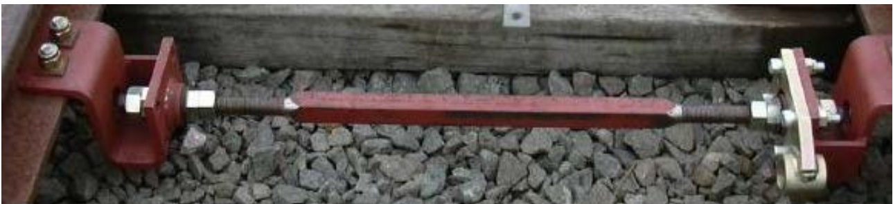
Figure 9 – Adjustable stretcher bar using hardlock nuts fixed to Shallow Depth Rail
