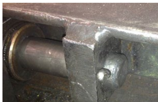
Figure 12 - Split Pins and Switch Rail Bracket Lugs
