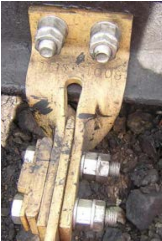
Figure 7 – Yellow stretcher bar bracket with hardlock fastenings
