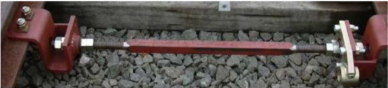
Figure 9 – Adjustable stretcher bar using hardlock nuts fixed to Shallow Depth Rail
