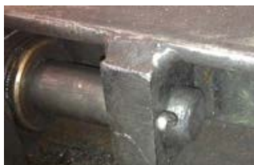
Figure 12 - Split Pins and Switch Rail Bracket Lugs
