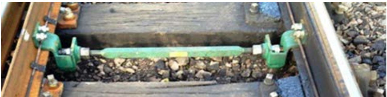
Figure 10 – Adjustable stretchers bar using hardlock nuts fixed to Full Depth Rail.
