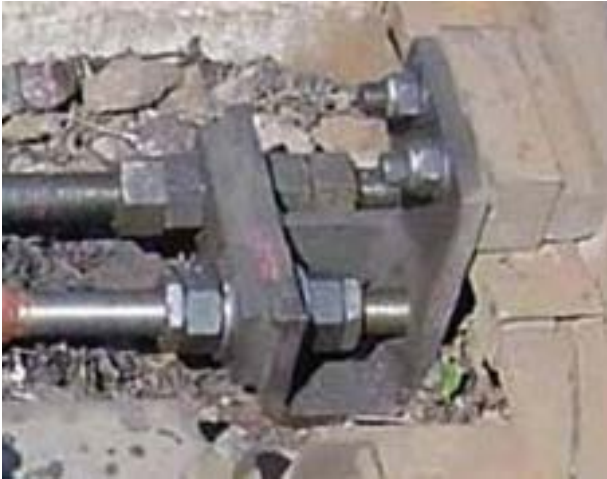
Figure 11 - Adjustable stretcher bar Mk. 1 bracket using half/full nuts (supplementary drive also shown).
