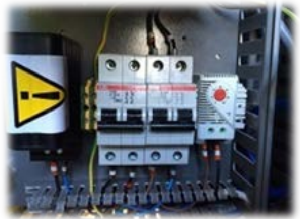
Figure 10 – Isolation MCB's
