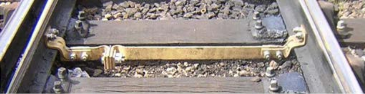
Figure 6 – Yellow fixed stretcher bar with hardlock fastenings
