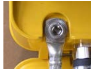
Figure 5 – Earthing point
