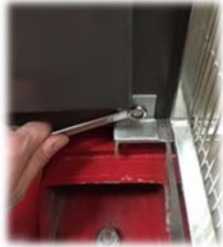
Figure 16 – M8 Side arm fixings
