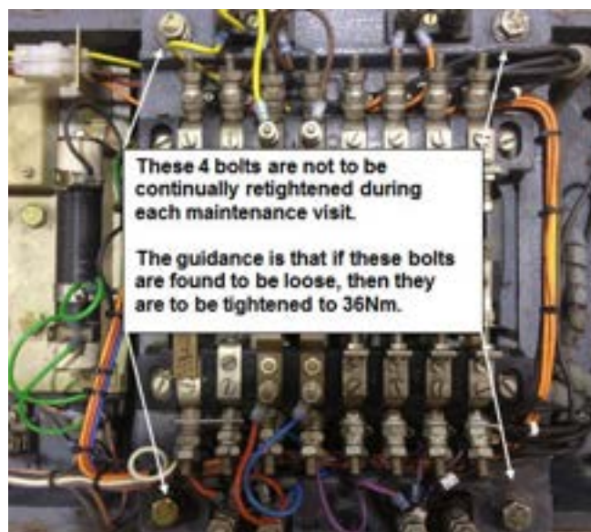
Figure 16 – Detection Frame bolts
