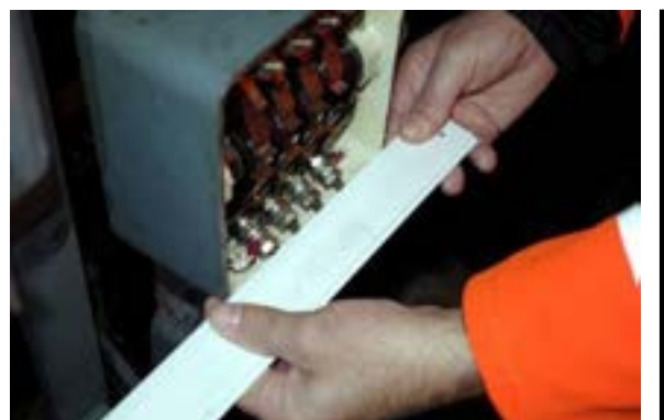
Figure 1 – Stud length check
