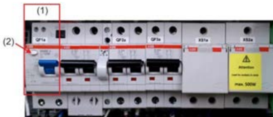
(1) Residual current circuit breaker. (2) Test button.
