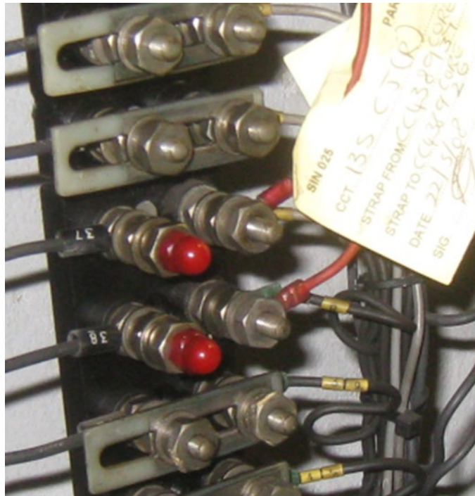
Figure 2 - Diversion Applied to a Terminal Block
