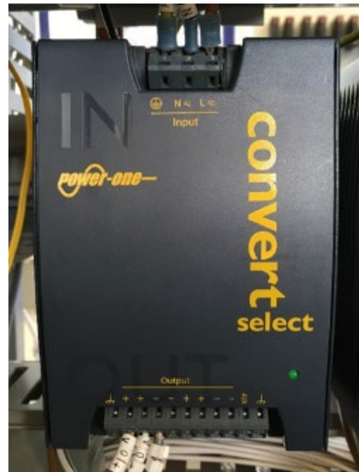
Figure 1 - Powerone AC-DC Converter
