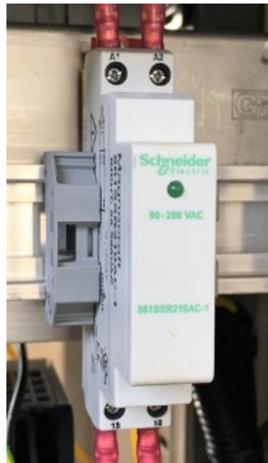
Figure 1 - Schneider Relay
