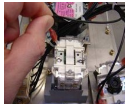
Figure 11 – Swapping Wiring to new contact block
