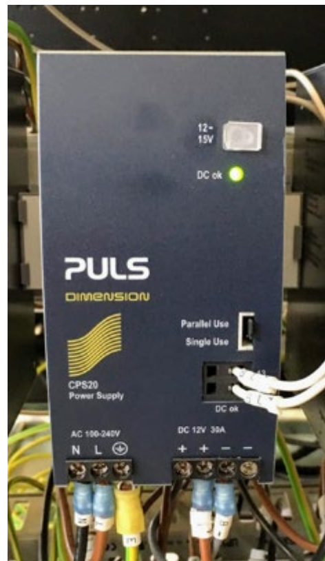
Figure 2 - CPS20.241 Power Supply
