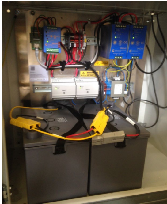
Figure 1 – Power Supply Module and Battery Pack
