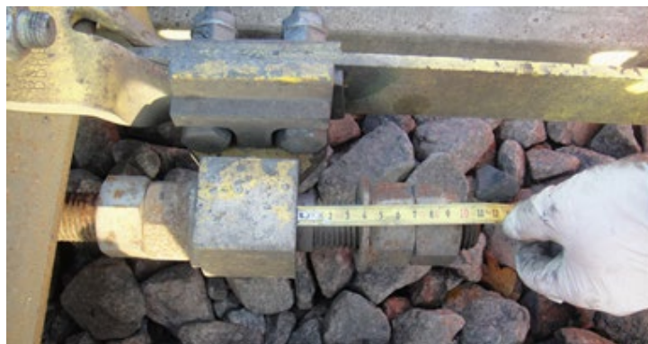
Figure 1 – Photo of Escapement Measurement
