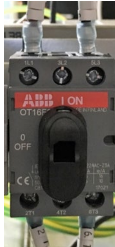
Figure 1 - ABB Power Switch OT16F3
