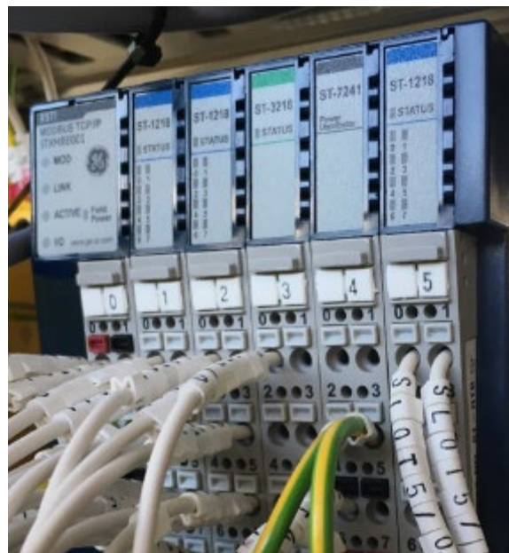
Figure 1 - Five RSTi ST Modules fitted to a TCP-IP Network Adapter
