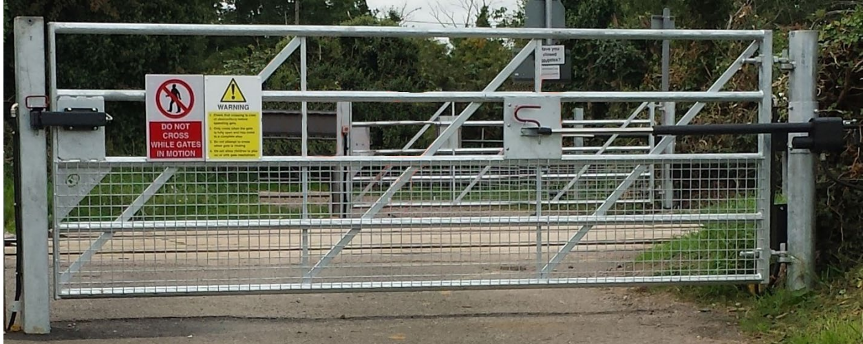
Figure 1 - NR2 - Power Operated Gate Opener (POGO)
