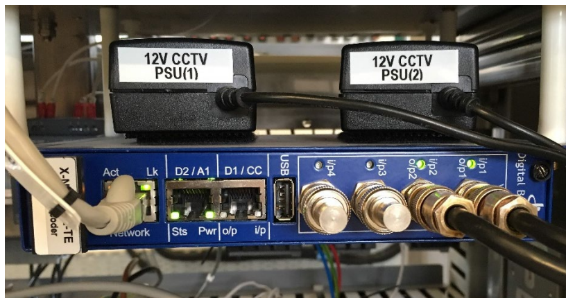
Figure 1 - X-Net Encoder PSU
