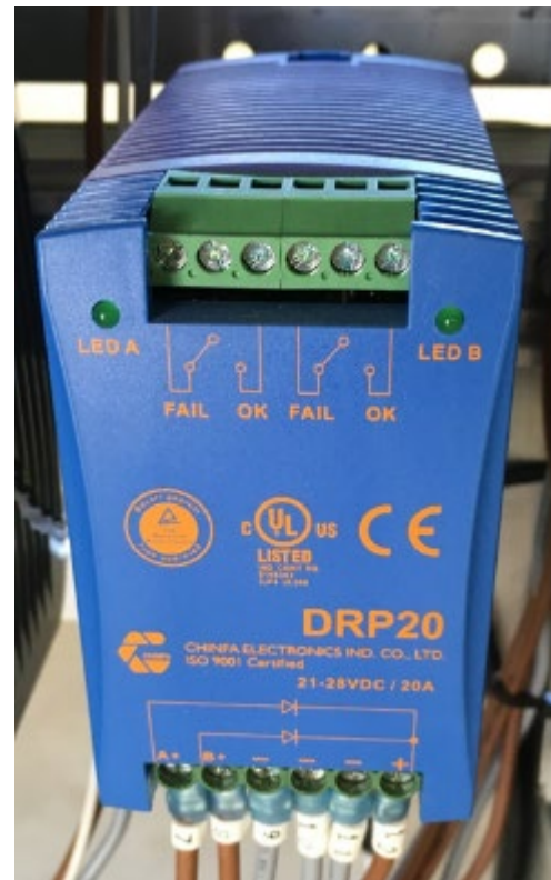
Figure 1 - CHINFA DRP20 Redundancy Unit
