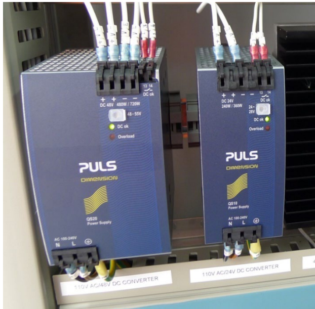
Figure 6 - AC-DC converters showing DC OK indication
