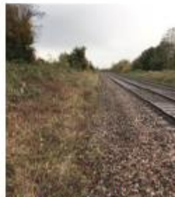
Figure 1: The planning of the safe system of work was undertaken in winter and based on a safe walking route due to minimal vegetation
