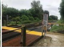
At this site - Sturry, neor Conterbury - the team removed the skew and the step up, thereby making the crossing safer for the public.
