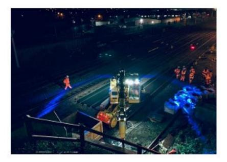
Recently, there have been many articles relating to lighting systems fitted to On Track Plant. These lights are blue lamps projecting beam patterns to depict exclusion zones on the ground. These systems have not been reviewed through the Product Approval process, and therefore should not be used.
