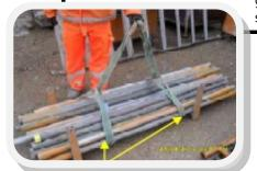
Weight of scaffold tubes secures frame during lift
