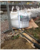
During the lowering of a one tonne sand bag a heras fence panel and / or the supporting foot was accidentally moved and damaged a nearby 750 volt supply positive feeder cable.
