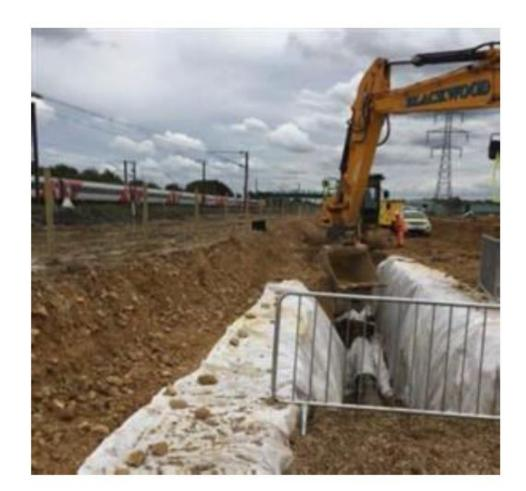
On 30th September during installation of drainage works, at Stamford Underbridge, a survey levelling rod was left in a trench by mistake. A trench box had been in use earlier but not when a supervisor entered the trench (2.5 – 3.0 metres deep) to retrieve the rod.
