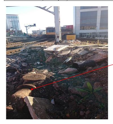
We came across this redundant steel pipe when we removed Platform 6/7. It heads in the direction of our dig so there is a possibility we may come across it whilst digging. The machine will have to pull it out if it comes across it. It is in collared sections so should come out if required.
