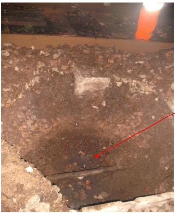
We exposed the pipe near the end of the platform and found it to be much deeper.
