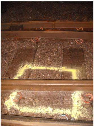
These photos highlight the redundant drainage chamber and its position under 821 points. This can be removed or filled in during the excavation.
