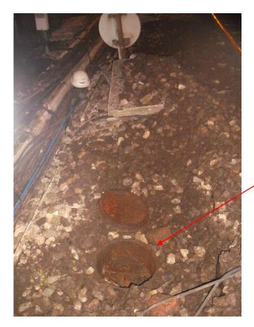
The pipe detailed on the previous page runs into this small circular chamber which we discovered. This can also be removed during the dig.
