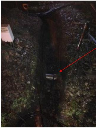
This clay duct crosses under the track near to the above ducts. It is a redundant service which ran through Platform 6/7. It runs into a small chamber which sits under 821 points.
