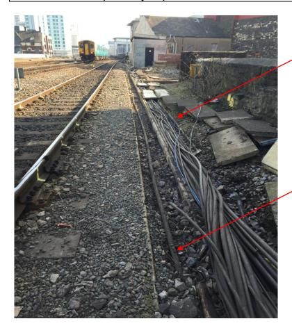
We have removed most of the dead cables from these trough routes and placed the remaining ones into the outer route so the inner trough route can be removed for the dig if required. There may be cables under the trough route but they will be dead.
