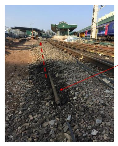
This small pipe runs through the ballast shoulder in the direction shown. It will be in the shoulder for the extent of the excavation so when it is exposed we can cut it with a disc cutter.
