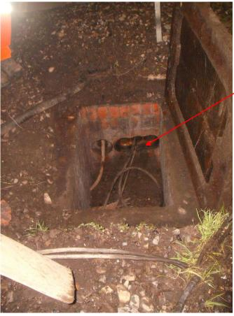
This chamber sits by C425 signal. The chamber itself appears to be out of the dig area but the cables inside it cross under the track at a depth shallow enough to suggest we will come across them whilst excavating. The cables are all dead so the excavator can either dig through them or we can cut them when exposed.
