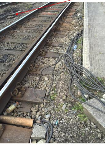
There are cables crossing under the track here which we have proved dead and cut. We believe that 2 of them emerge in the route which is visible here.
