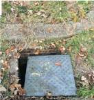
An operative working for the supervisory controls project sustained a leg injury whilst surveying external cable routes at Penge sub-station. As he walked in an area covered in leaves, he stood on a cable chamber manhole cover which gave way beneath him. One of his legs plunged down the chamber to waist depth resulting in an injury to his right knee. He was taken to hospital where it was confirmed he had suffered serious ligament/tendon trauma, bruising and fluid accumulation to his knee.
