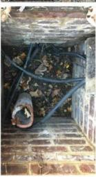
The manhole cover was refitted, tested and found to be in good condition. It transpired that the manhole cover had not been fitted properly by previous users which resulted in the cover not being seated correctly in its frame. This caused it to tilt when weight was applied. This accident was recorded as an over seven day RIDDOR event.
