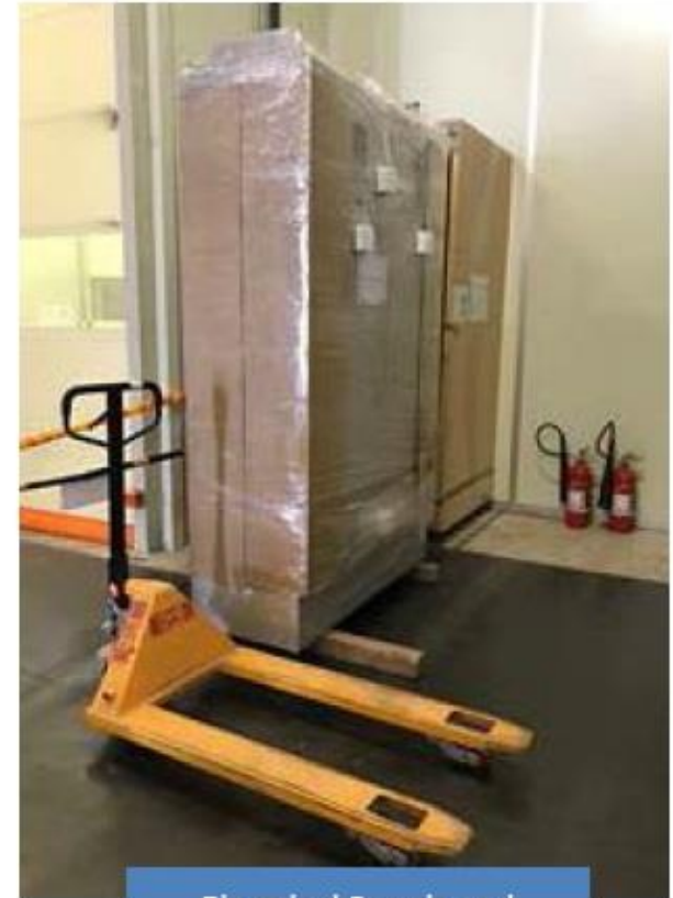
Electrical Panels and Pallet Jack
