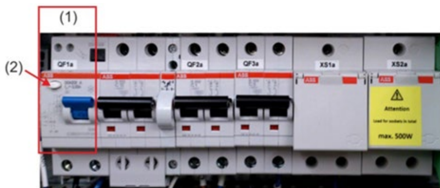
(1) Residual current circuit breaker. (2) Test button.
