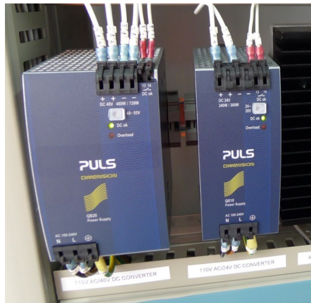
Figure 6 - AC-DC converters showing DC OK indication
